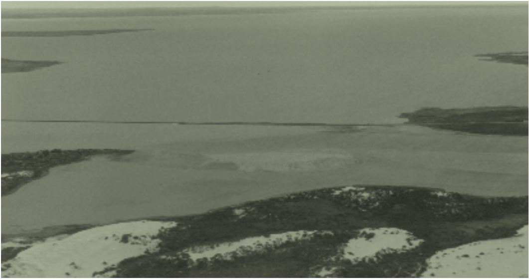
Tauwitchere Barrage no.(1) (2004)
