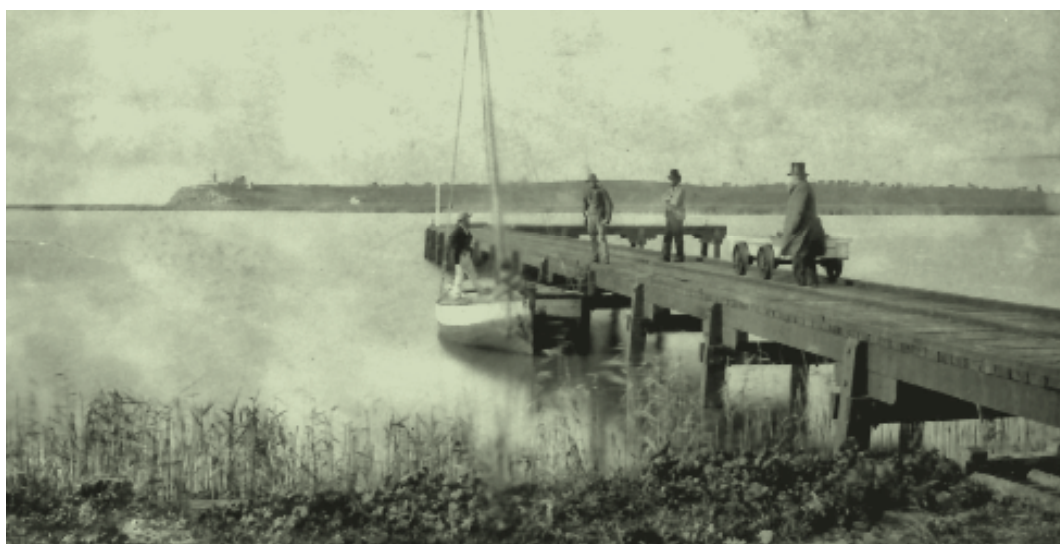
Jetty at Narrows between Lakes Alexandrina and Albert 1870s
