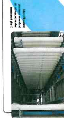
Advanced ultrafiltration membranes are used to filter out the smallest particles, including Micro Bacteria.
