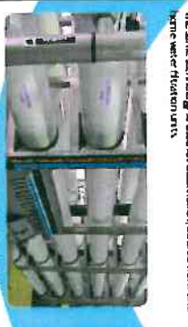
Reverse osmosis membrane filtration process.
