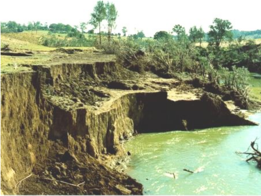
Photo 1: Badly eroded Mary River Banks after the 1992 flood
