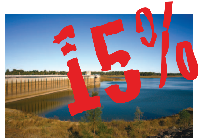
North Pine Dam
