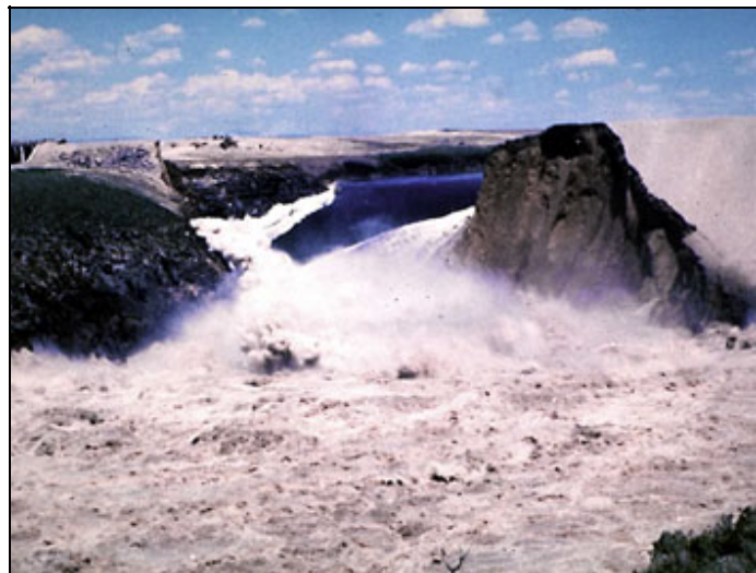
Teton Dam Disaster 1976, someone pulled the plug out.
