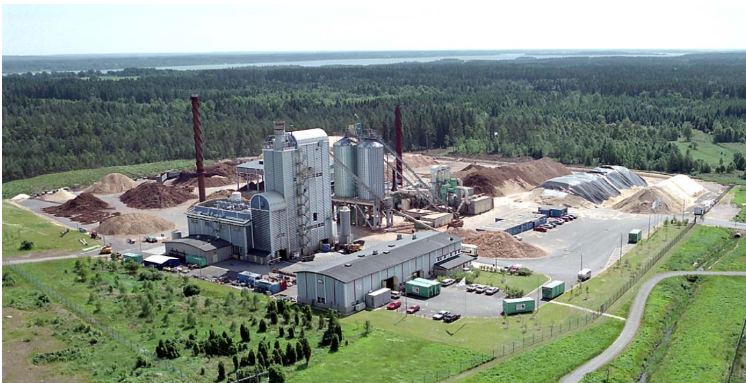
Figure 8 : Värnåmo BIGCC plant, Sweden
