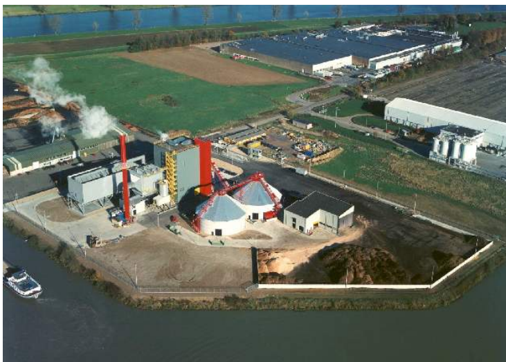
Figure 3: Aerial Photo of Cuijk 25 MW power plant (source Essent Energy)
