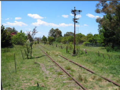
Rehabilitation rural rail lines
