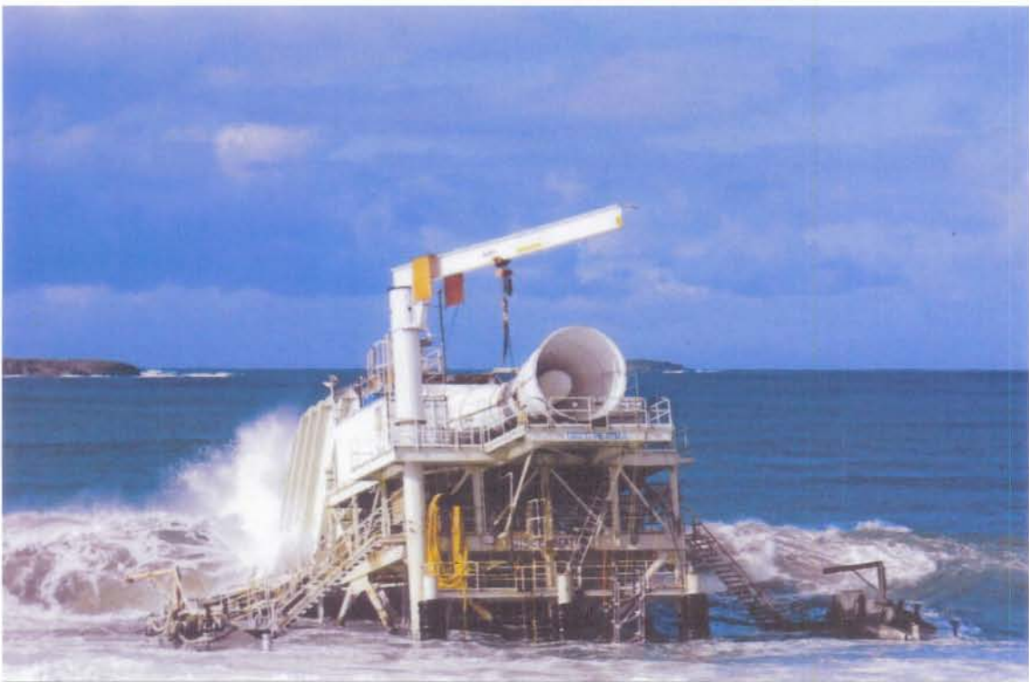
The wave power demonstration plant at Port Kembla, developed and tested locally by Tom Dennis at Oceanlinx.
