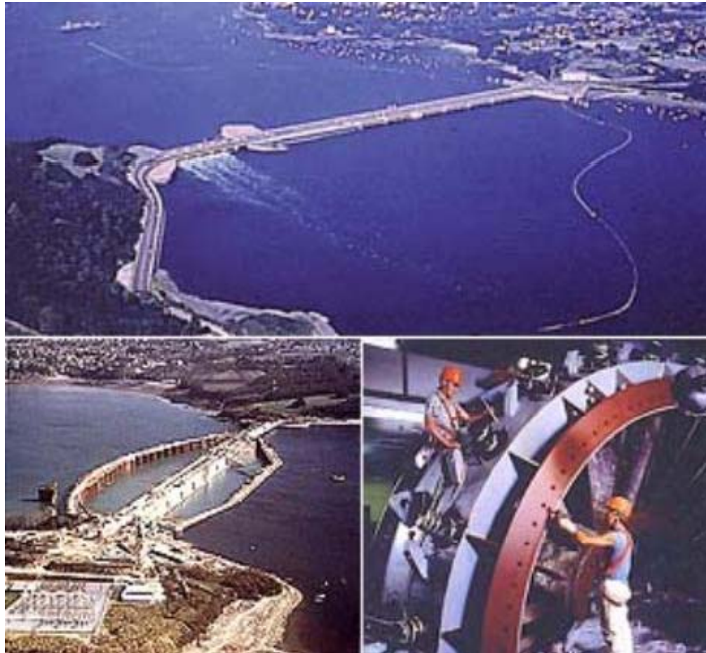
Source (2): La Rance Tidal Power Station during and after construction (Image courtesy of Popular Mechanics).
