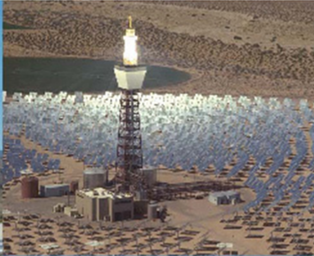
Heliostat field with power tower
