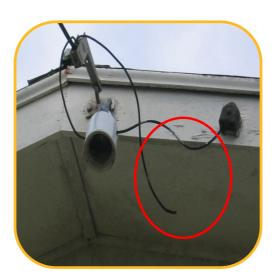
Examples of faults detected in Tasmania – Degraded Active If left un-detected, these faults have the potential to lead to house fire and will certainly lead to service disruption.
