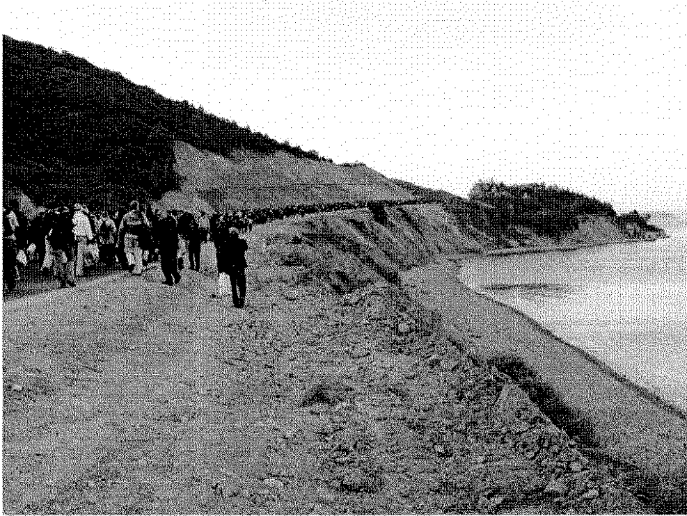
Fig 5 - Road construction adjacent to ANZAC Cove has greatly altered the foreshore line and the "sense of place"
