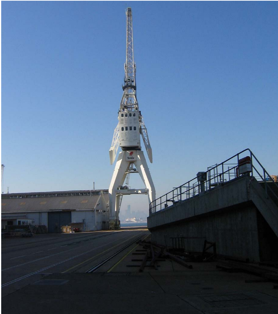
The Tenix Williamstown 64 tonne slipway crane
