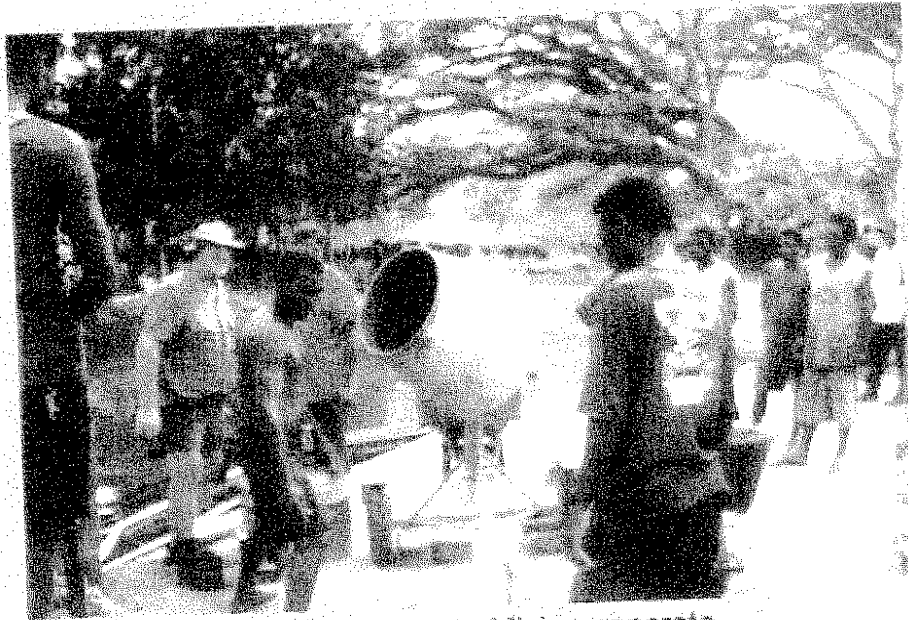
Maravovo Ford - Mixing concrete.
