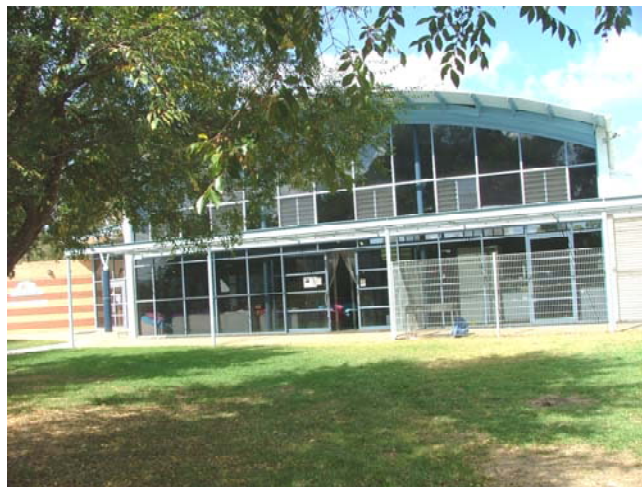
HANGAR BUILDING – WODONGA CAMPUS
