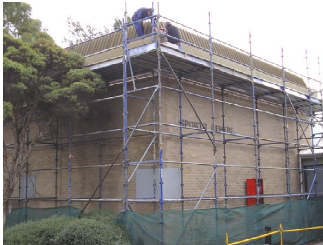
SPORTS CENTRE UNDERGOING REPAIRS (COSTING $27,000) – BUNDOORA CAMPUS
