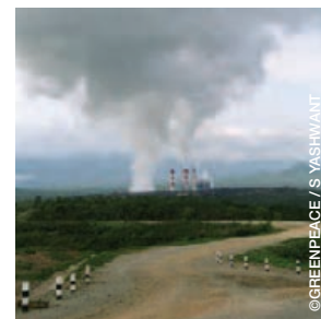
image Smoke stacks of the lignite (brown coal) fuelled Mae Moh power plant discharging smoke, Mae Moh, Lampang province Thailand.
