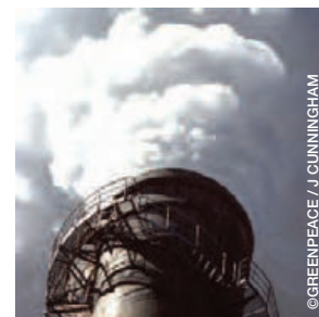
image Cementa cement factory, Gotland, Sweden.
