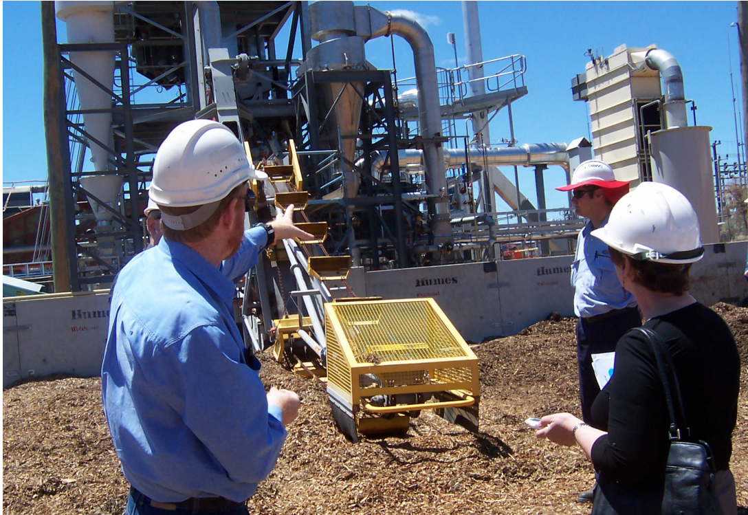
Photograph: the Integrated Wood Processing Demonstration Plant, Narrogin, WA
