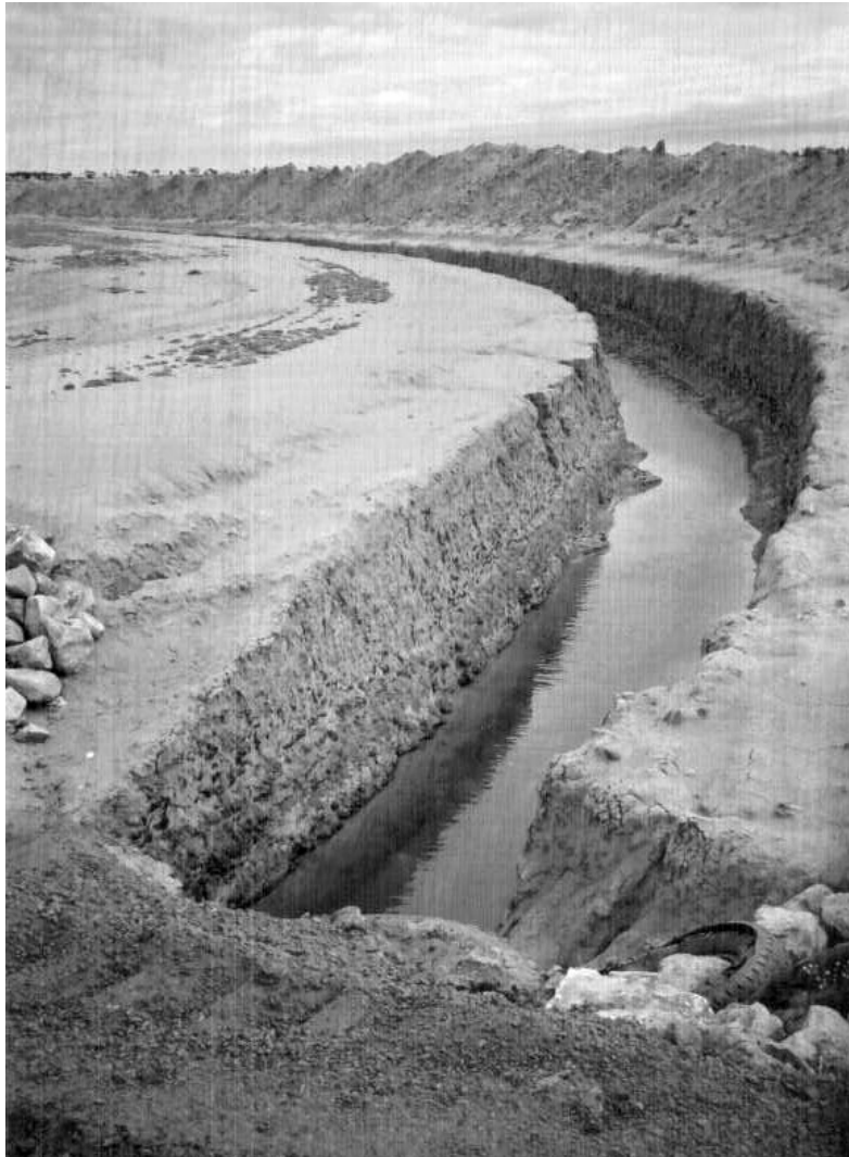
Photograph: Gents-Trayning deep drainage site, WA
