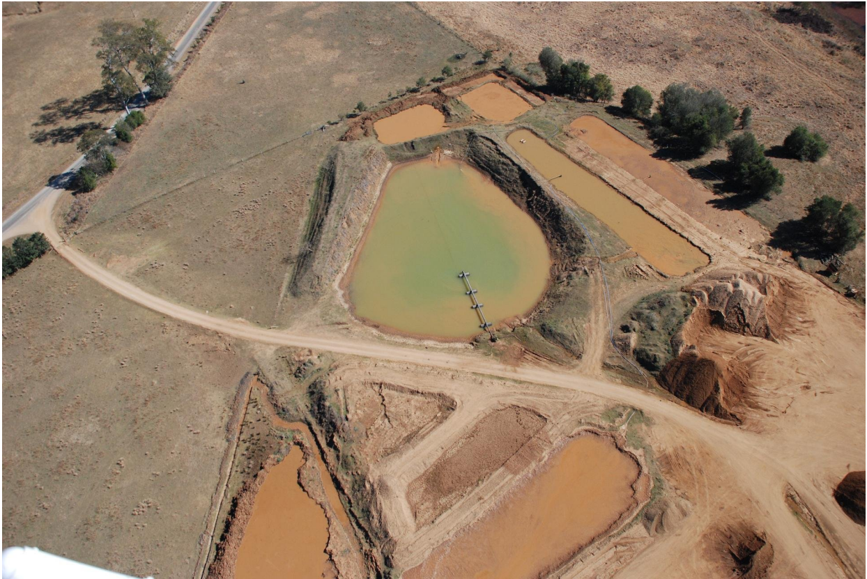
Photo 2: Closer view of highly dispersive silts in settling ponds in the flood plain at Traveston Crossing. There exists a high risk that these will be breached during a high flood event. Aug 2008.
