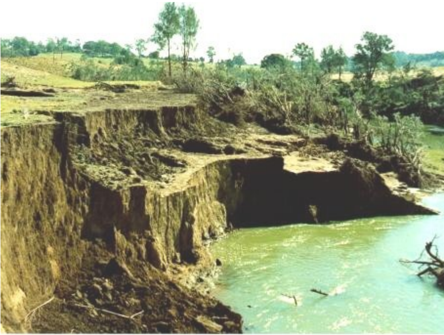
Photo 3: Badly eroded Mary River Banks after the 1992 flood
