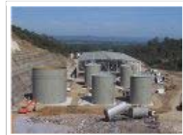
WSN's Macarthur Resource Recovery Park
