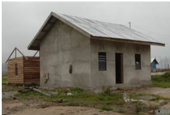
A new Habitat for Humanity home under construction
