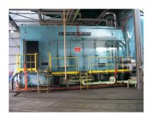
A ProtxL Filter Module fitted to a 100meg turbine removed moisture and particulate contamination and maintained oil cleanliness to better than NAS 6 Standard. ProtxL will maintain TBN and control the TAN in the oil and also has proven that clean dry oil reduces vibration within the turbine.
