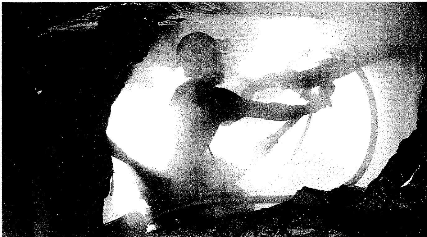
02 Rock drilling workers are exposed to the dust almost daily.
