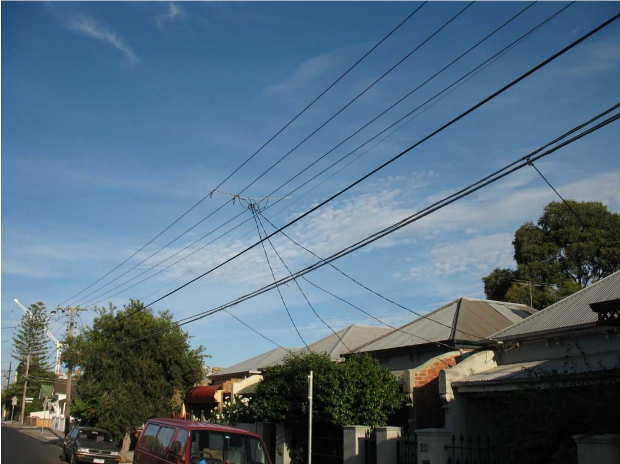
Figure 1: Existing mid-span lead-ins providing electricity and pay television services in Brunswick, Victoria to narrow frontage properties.
