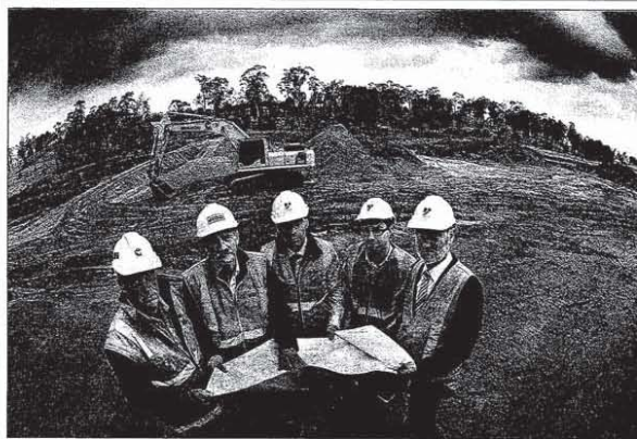
Gradco project supervisor Rodney Grace, Dale Luck, of JMG Engineers, Launceston City Council infrastructure director Harry Galea, council graduate engineer Josh Coates and Mayor Albert van Zetten at the Mount Pleasant Dam site.
