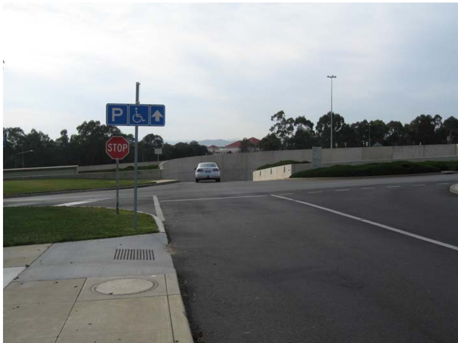
Photograph 6 – Lack of pavement arrows to assist motorists with available options
