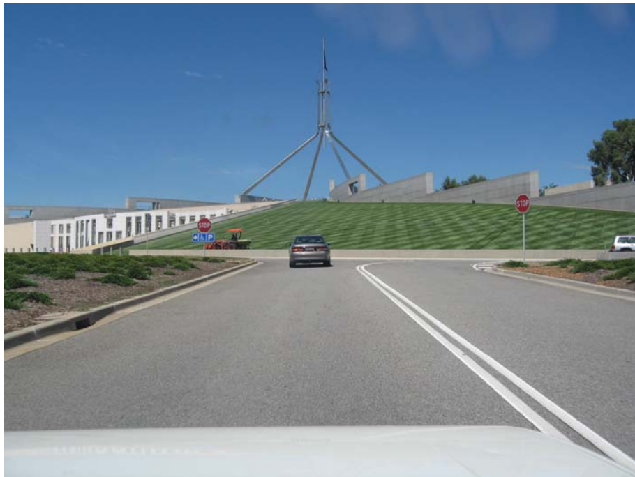
Photograph 7 – Commonwealth Avenue approach to Parliament Drive where motorists turning left are required to stop unnecessarily
