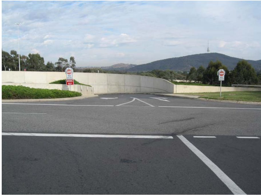
Photograph 5 – Misleading linemarking at public car park exit
