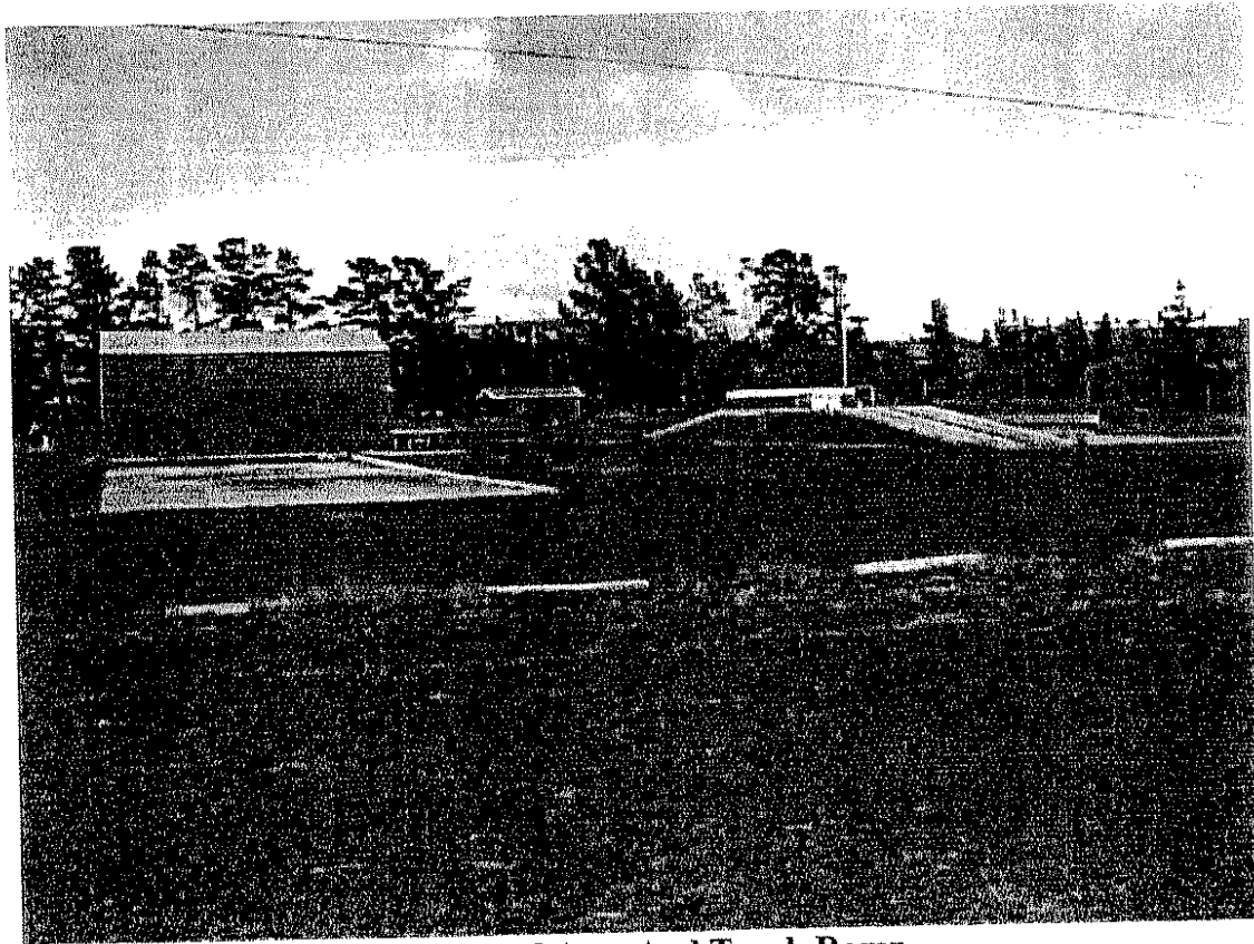
Hardstand Area And Truck Ramp
