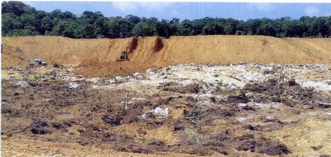
Earthworks underway at mine field 20E in October 2004
