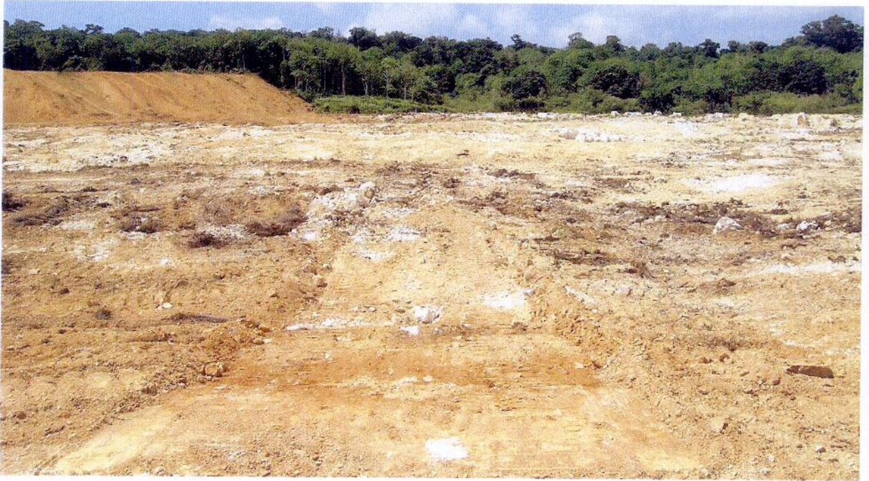
Figure 5: Mine field 20E cleared, pinnacles flattened, and the stockpile face cleared ready for soil loading and haulage.
