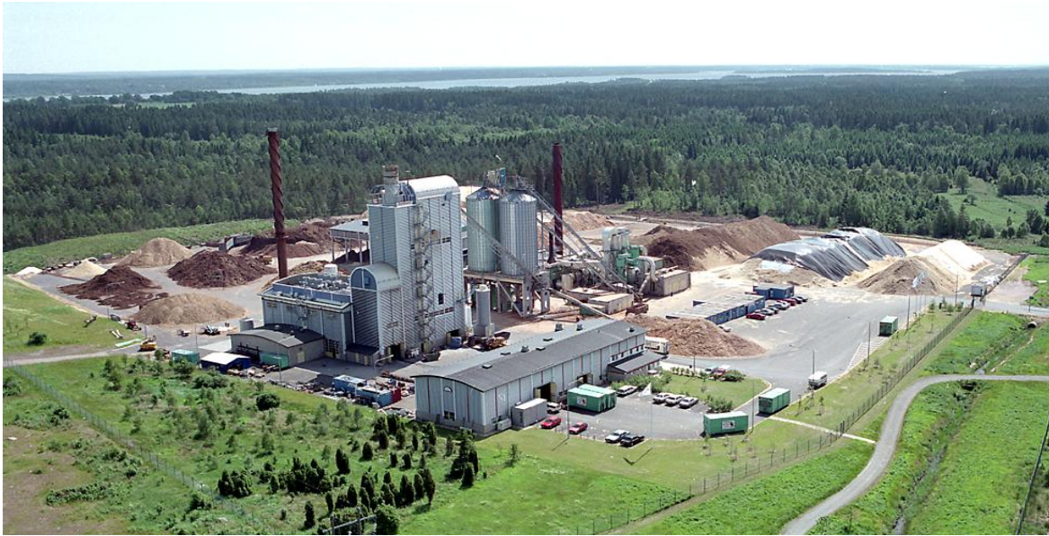
Figure 12 : Värnamo BIGCC plant, Sweden
