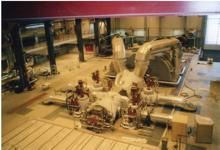
Figure 10: Alholmens Kraft Turbine Hall Showing 240 MW Steam Turbo-Generator
