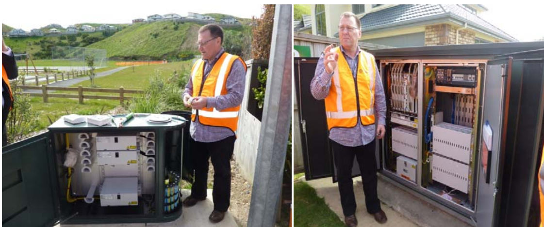
NZ Figure 5 A Chorus representative showing the cabinet infrastructure supporting the copper and fibre networks
