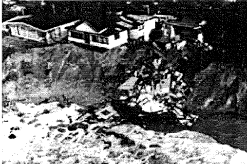
Figure 3: Wamberal property damage in 1978 due to beach erosion
