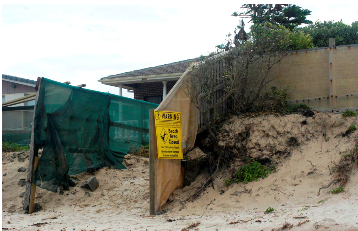
Example of coastal dune erosion, North Entrance, Central Coast, NSW—see Submission 5
