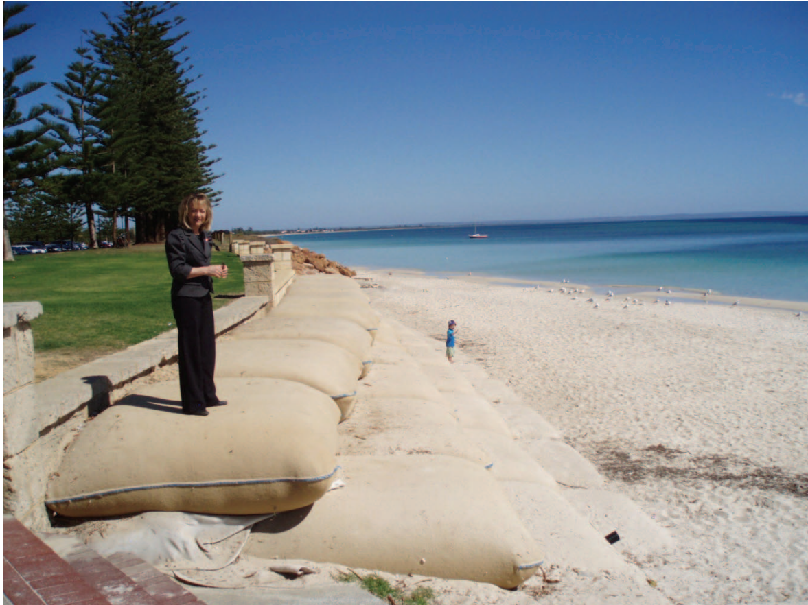
Foreshore protection at Busselton, WA, as inspected by Committee members
