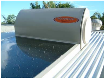
Solar hot water is one option for heating water for guest cabins.
