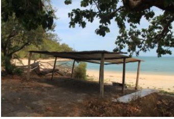
Existing shack, Mutee Head.
