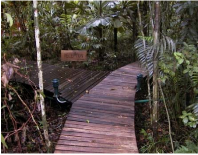
Timber boardwalks between huts and the main buildings can be used to carry sewage, water and power supplies.
