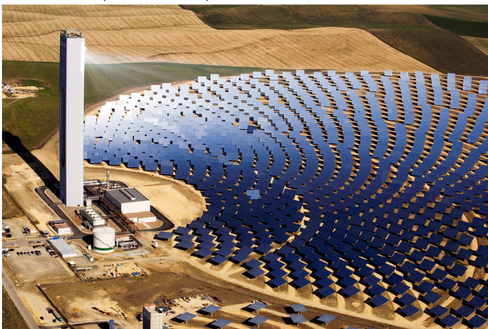
Figure 5. Example of an operating solar thermal power plant in Spain, which uses solar power tower technology (Image: Greenpeace).
