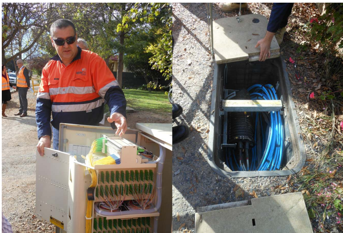
Figure 5.1 Inspection of Willunga, South Australia
