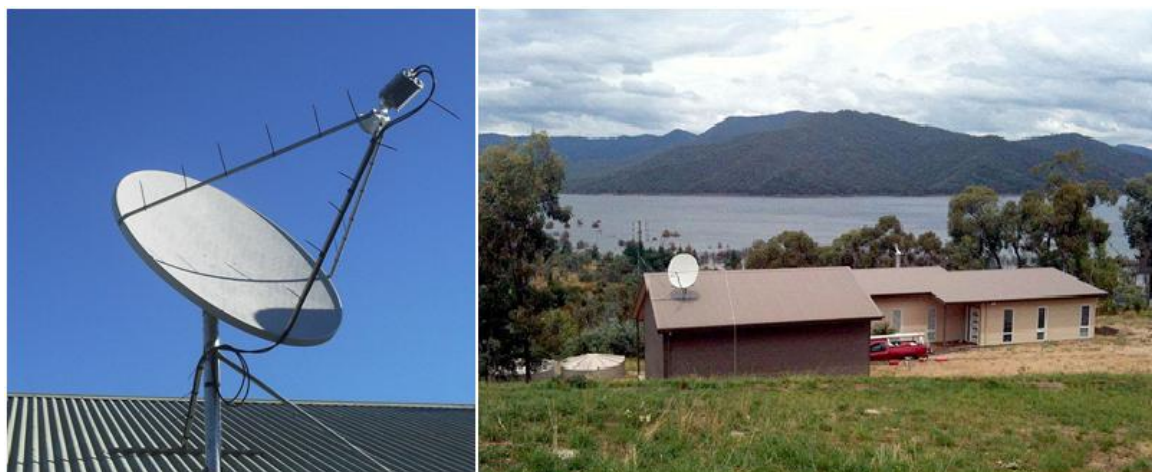
Figure 5.4 Roof-mounted National Broadband Network Satellite Receiver
