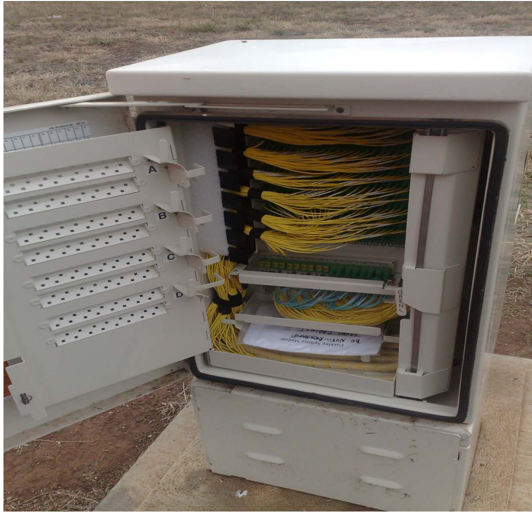
Fibre Connect Cabinet
