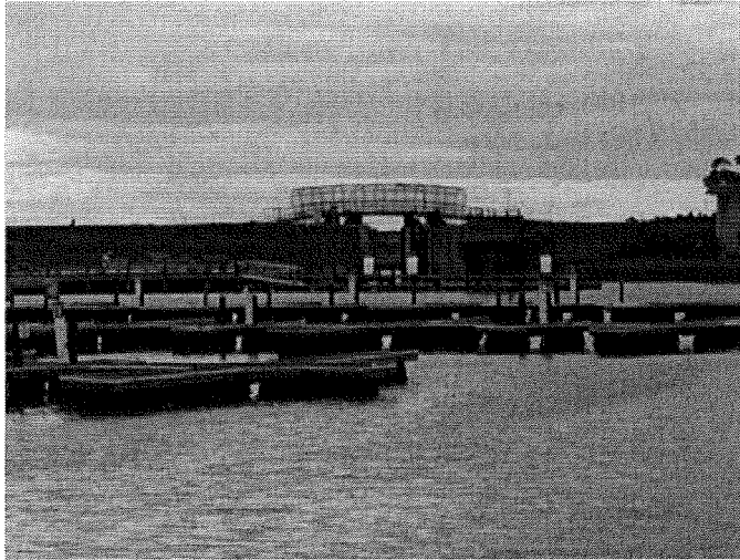
Fig 3. Canal estate with flood protection – Patterson Lakes, Victoria (Photo by N Farmer)
