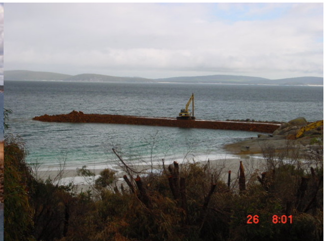
BREAKWATER UNDER CONSTRUCTION 26/10/05
