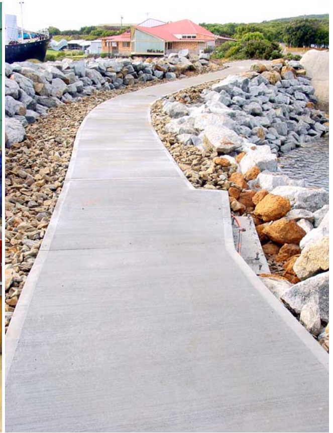
CONCRETE PATHWAY COMPLETED 16/2/06
