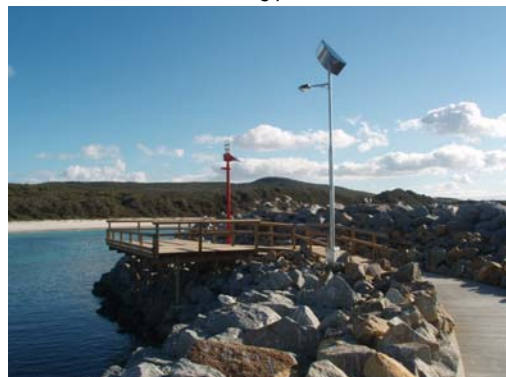
Safe fishing platform with solar-powered night lighting
