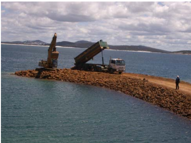
BREAKWATER UNDER CONSTRUCTION 28/10/05
