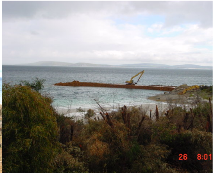
BREAKWATER UNDER CONSTRUCTION 26/10/05
