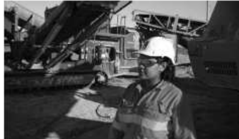
Narassa, Northern Project Contracting, on site at Century Mine in the Gulf of Queensland
