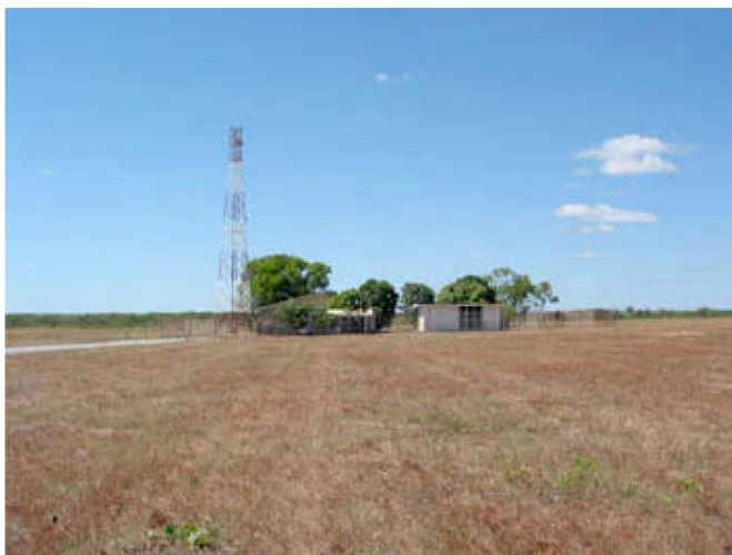
Photograph 1. Existing Receiver Station buildings.
