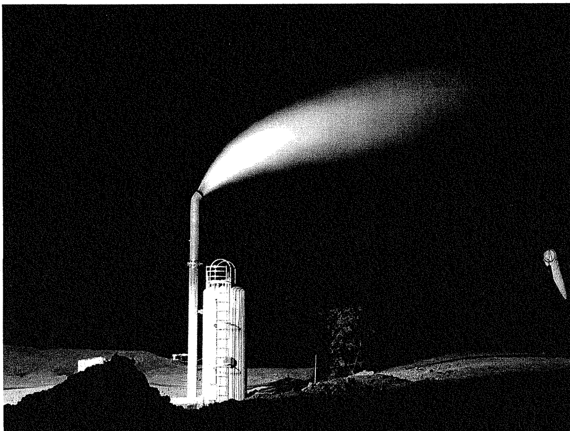
Figure 7. Small production test from Habanero 2. Note that in commercial production the geo-fluid will always remain as super heated water in a closed system, and never become steam.
