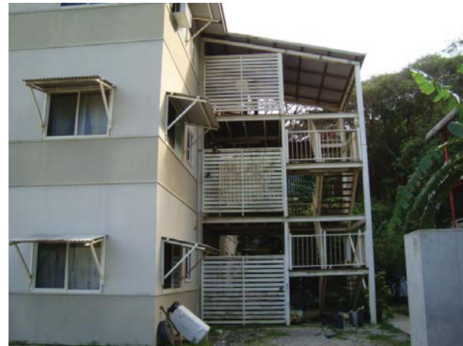
Low window to wall ratio, presents a building which is more institutional than residential. min overhang - screens filthy
