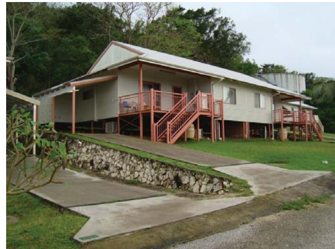
Relatively low window to wall ratio, means that dwelling does not interact with street, and exposed under floor unattractive
