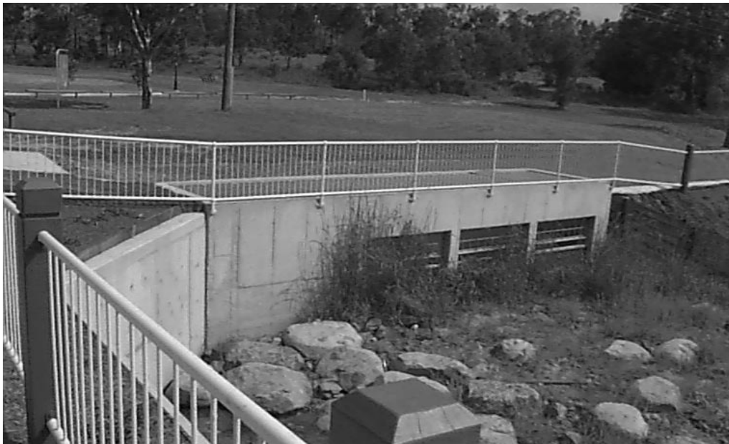
Plate 2 – Stormwater Quality Improvement Device
