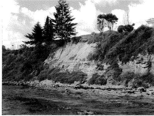
Cliff collapse Culburra Beach
