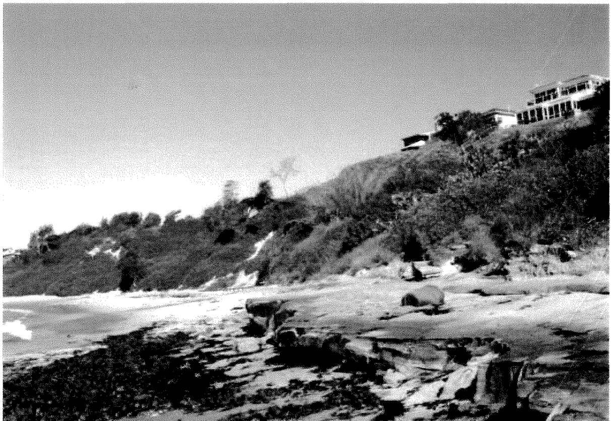
Photo from 1995 showing soil slippage.
