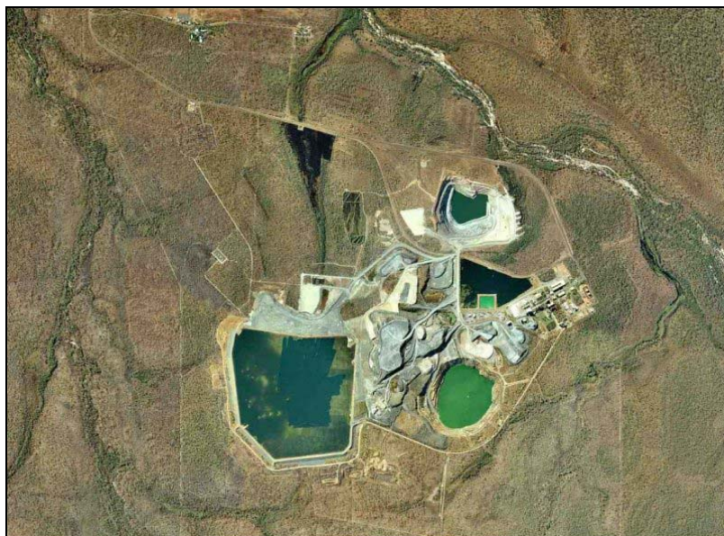
Figure 2.1 – Site plan of the Ranger uranium mine and mill and associated facilities 48 and aerial photo 49 (7 July 2001) [Note : RP4 is now decommissioned.]
