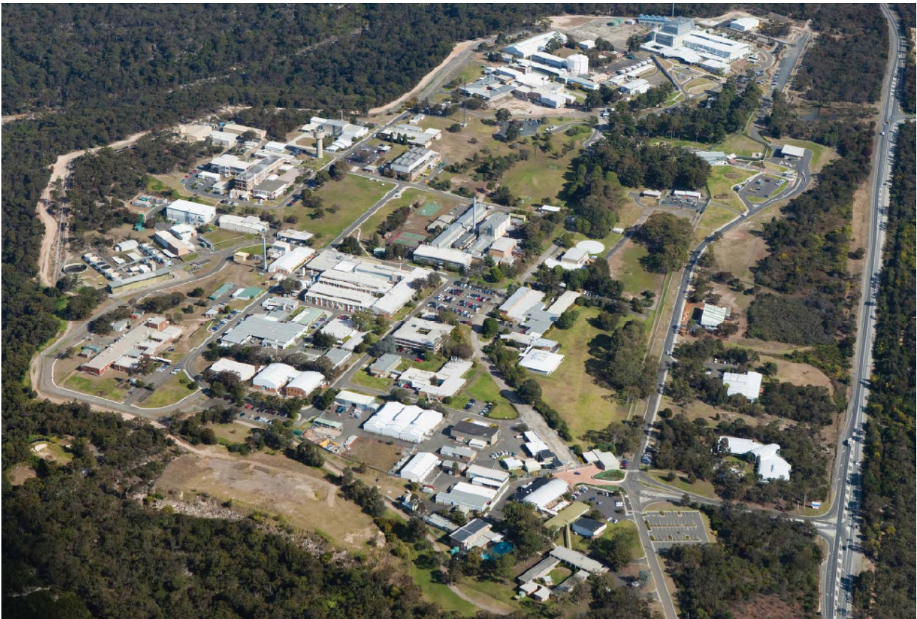
Figure 2: Aerial view of the ANSTO site taken from the North East
