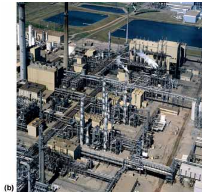
Figure TS.4. (a) CO 2 post-combustion capture at a plant in Malaysia. This plant employs a chemical absorption process to separate 0.2 MtCO 2 per year from the flue gas stream of a gas-fired power plant for urea production (Courtesy of Mitsubishi Heavy Industries). (b) CO 2 pre-combustion capture at a coal gasification plant in North Dakota, USA. This plant employs a physical solvent process to separate 3.3 MtCO 2 per year from a gas stream to produce synthetic natural gas. Part of the captured CO 2 is used for an EOR project in Canada.
