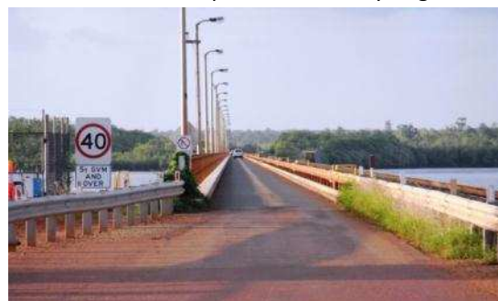
Rio Tinto road and rail bridge Weipa
