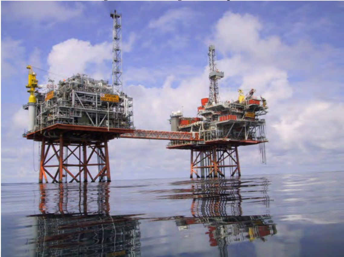
Photo 1 Offshore Integrated Deck - Large and Complex 1
